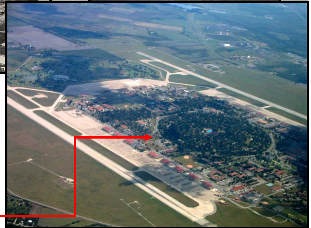
Historic District Base Housing Area
